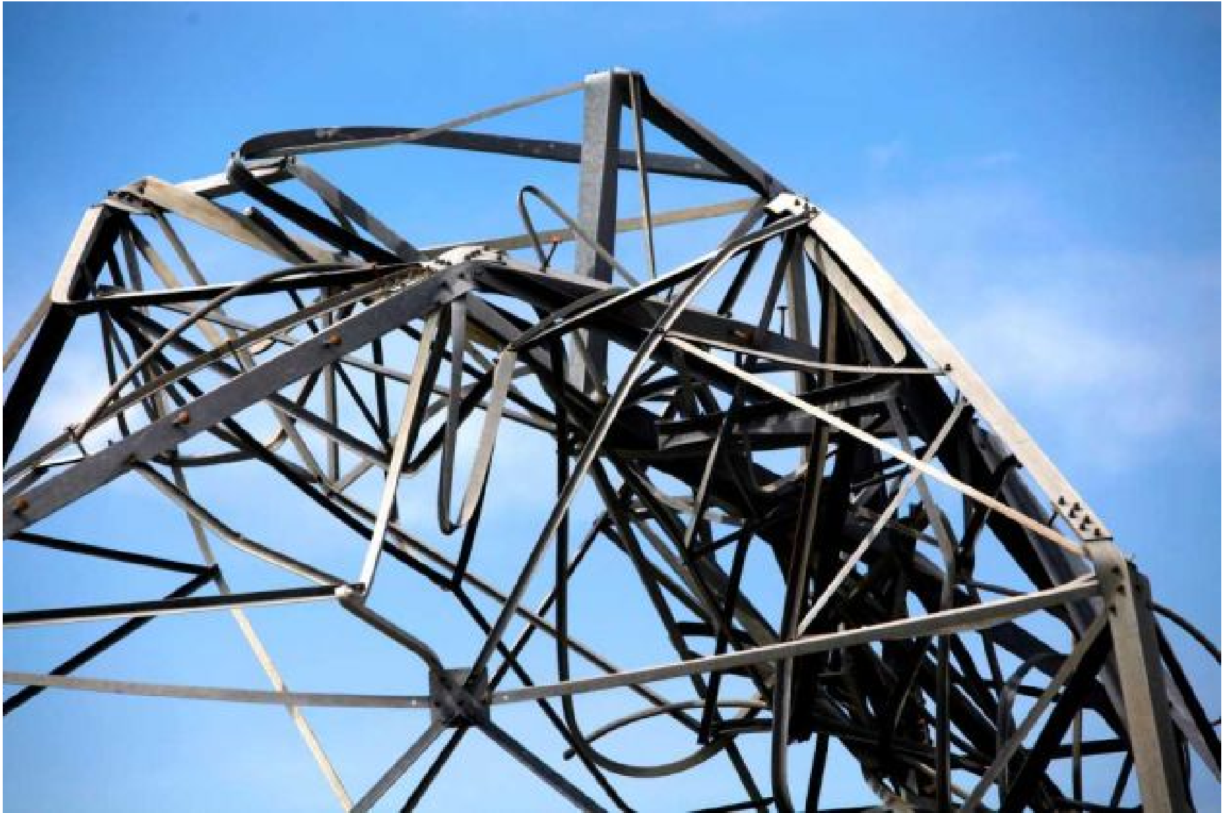
Collapse of towers for transmission lines
