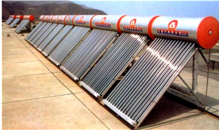
Fig. 2. Water-in-glass solar water heaters in China.
