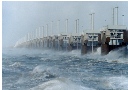
Figure 10.4: The Oosterscheldekering, a series of dams and storm surge barriers to protect the province of Zeeland from flooding from the North-Sea. Photo by Rijkswaterstaat, 2007, taken from Beeldbank Rijkswaterstaat , under BY-NC license [28].
