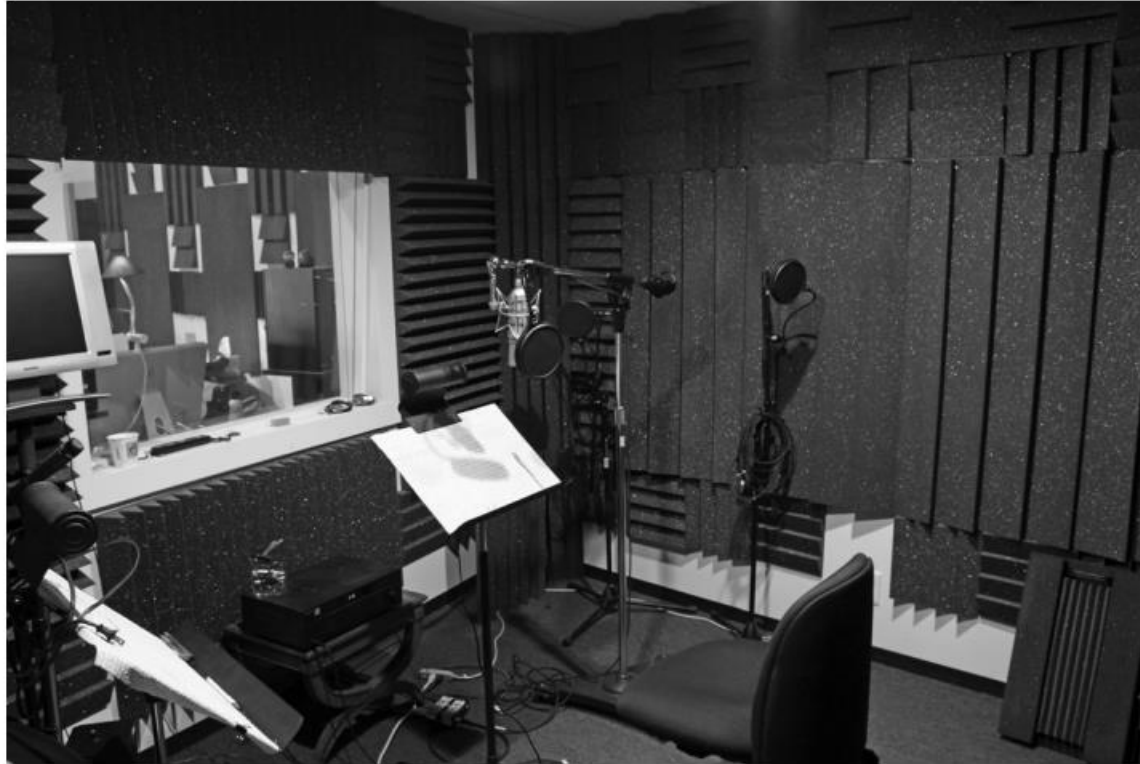
Figure 8.2 A dead room has absorptive surfaces that minimize reflections. (Sky Recording, Kansas City, MO).
