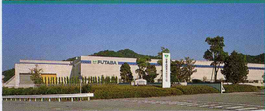
FUTABA INDUSTRIES SATTA PLANT 6DK-28 1500kW×2
