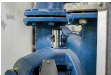
A pump fitted with a Machine Sentry sensor.
