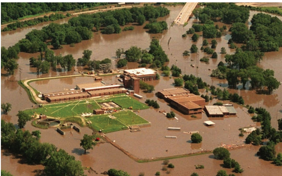
▶ FIGURE 10.22 Flooding during the summer of 1993 covered a vast area of the upper Midwest. Here, floodwaters near downtown Des Moines, Iowa, during July, 1993, inundate buildings of the Des Moines waterworks facility. Flood-contaminated water left 250,000 people without drinking water.
