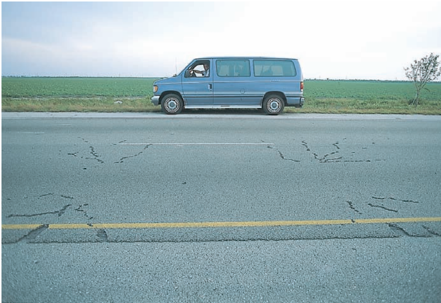
FIGURE 10.32 The four marks on the road surface represent areas where lightning, after striking a car traveling along south Florida's Sunshine State Parkway, entered the roadway through the tires. Lightning flattened three of the car's tires and slightly damaged the radio antenna. The driver and a six-year-old passenger were taken to a nearby hospital, treated for shock, and released.
