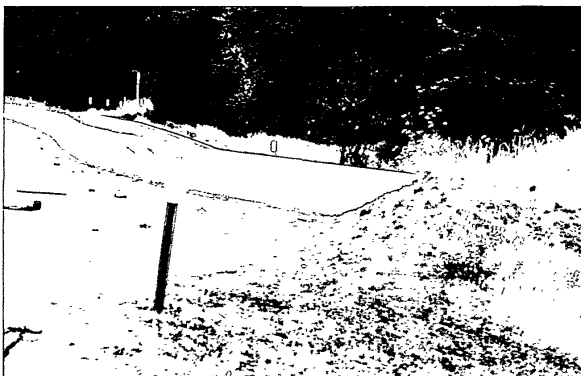
FIGURE 8.15 Barrier Anchored in Backslope
