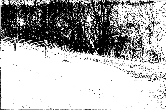
FIGURE 8.12 3-Strand Cable Terminal
