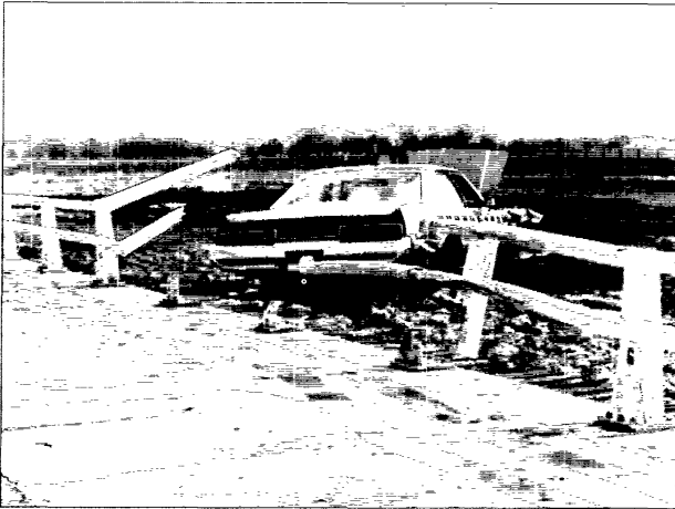
FIGURE 7.2 Inadequate Railing Strength
