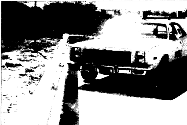
FIGURE 7.16 BR-1 Type C Aluminum Bridge Railing
