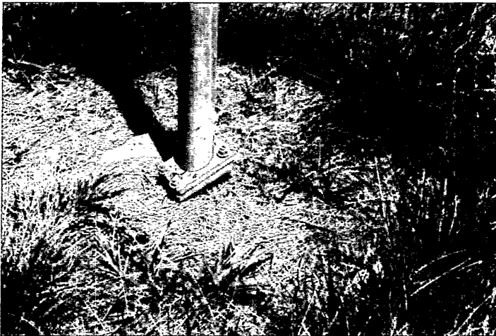
FIGURE 4.8 Uni-Directional Slip Base for Small Signs
