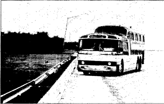
FIGURE 6.5 Self-Restoring Median Barrier
