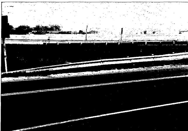
FIGURE 8.7 Turned-Down Guardrail Terminal
