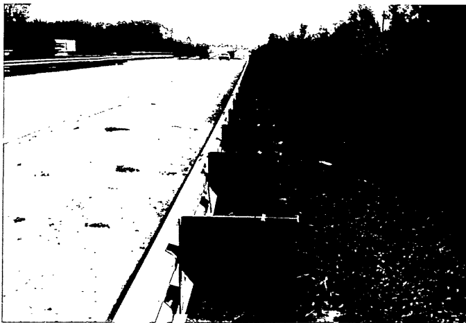
FIGURE 5.11 Modified Thrie-Beam Guardrail
