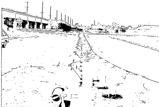
FIGURE 5.12 Self-Resting Barrier (SERB) Guardrail
