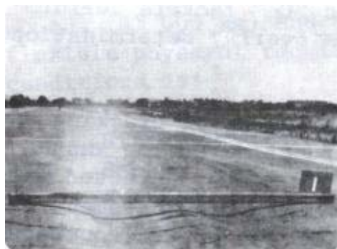
SURFACE OF OVERLAY
