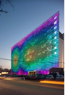
Greenpix Zero Energy Media wall: The largest color **LED display** combined with a **PV-system** in the **glass curtain wall**
