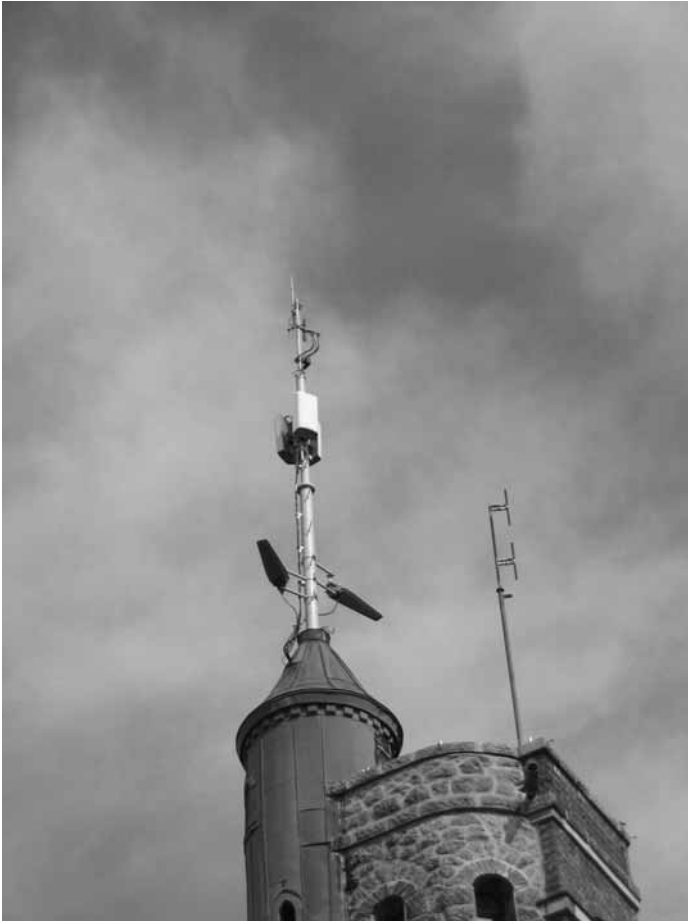
Fig. 31.38. Practical example of a translator or gap-filler site; the 2 (log periodic) receiving antennas are located in the lower part of the extended pinnacle of the tower, the 3 transmitting antennas (8-element bays) are located in its upper part
