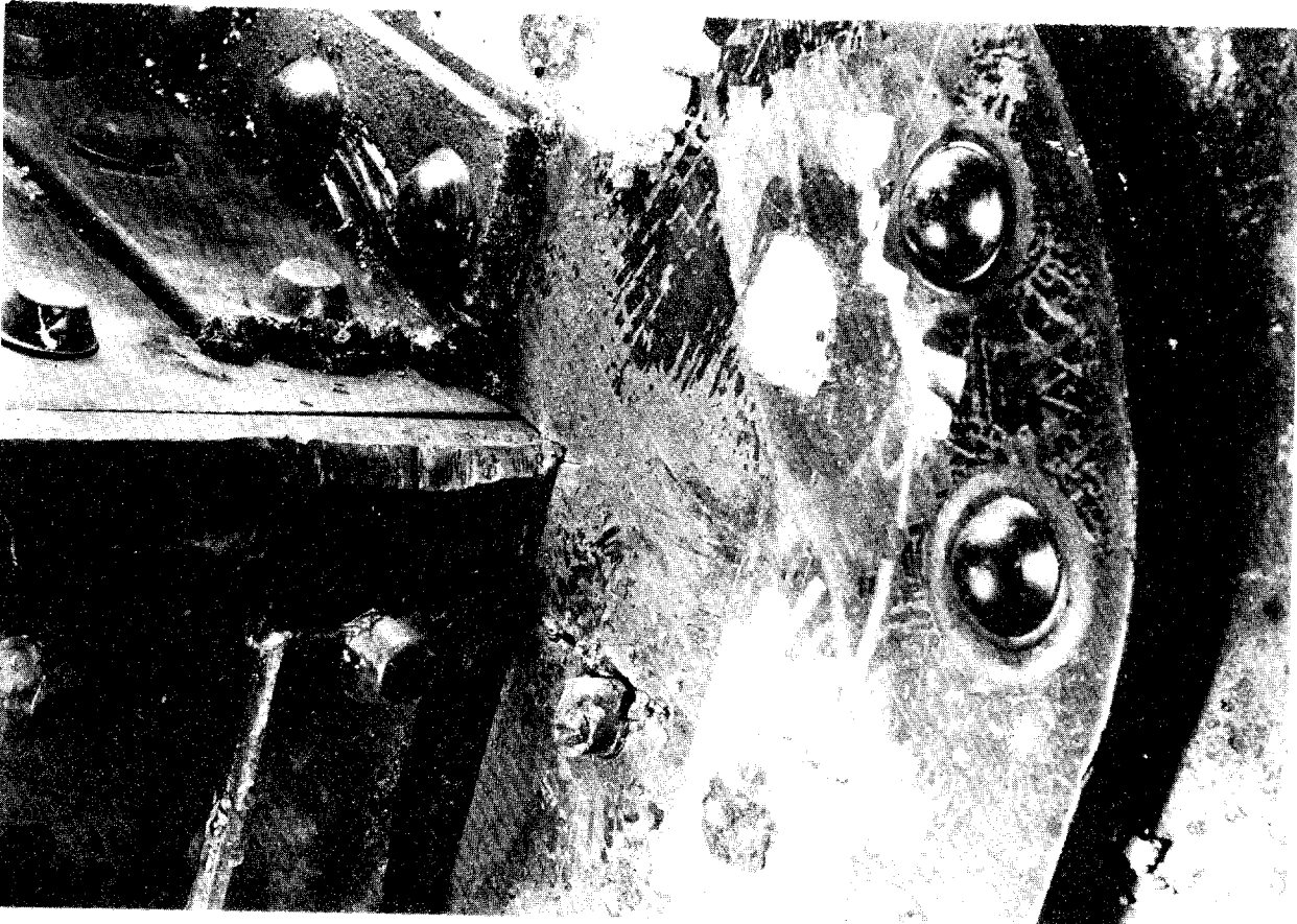
Fracture in Doubler (angle cut away)
