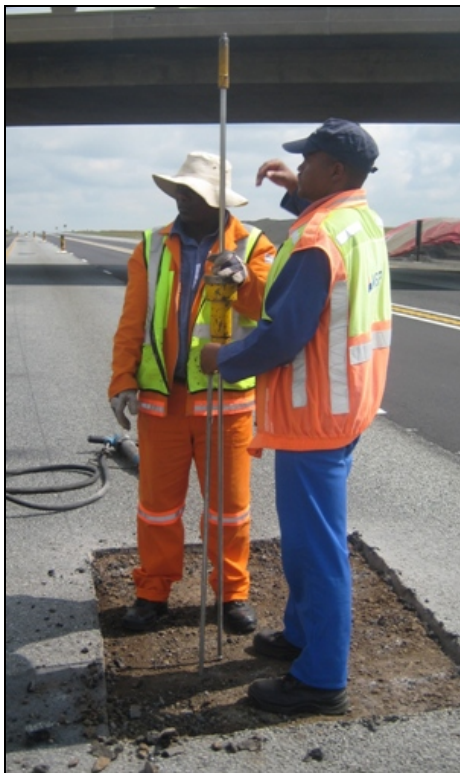
Figure 38. Dynamic Cone Penetrometer (DCP)
