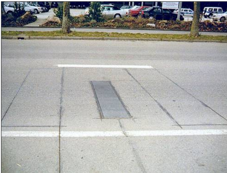
Figure 20. Typical WIM setup
