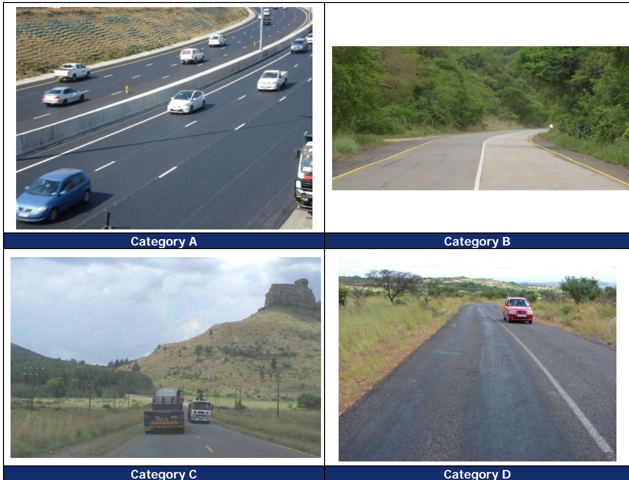
Figure 5. Typical South African Roads for Road Categories
