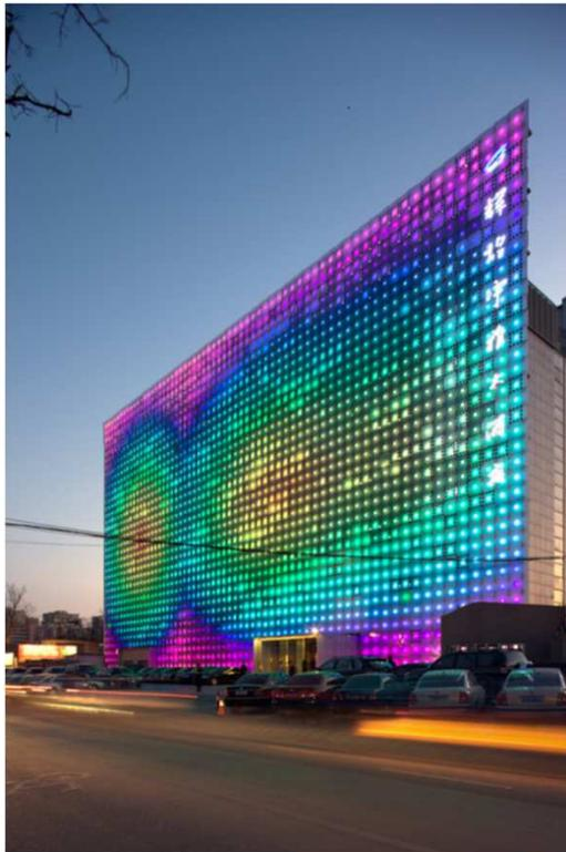
*Greenpix Zero Energy Media wall: The largest color LED display combined with a PV-system in the glass curtain wall*
