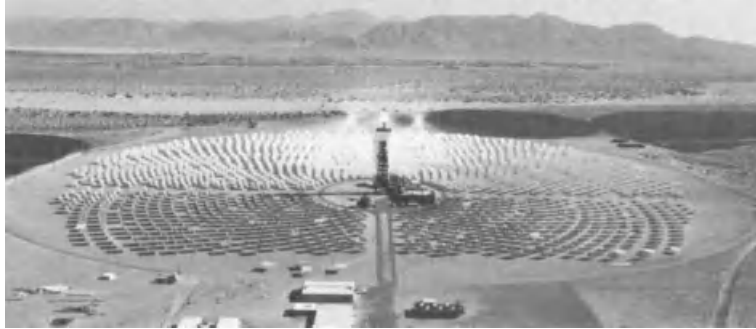
Figure 7.15.1 Solar One, a central receiver collector system. Photo courtesy of Sandia Laboratories.
