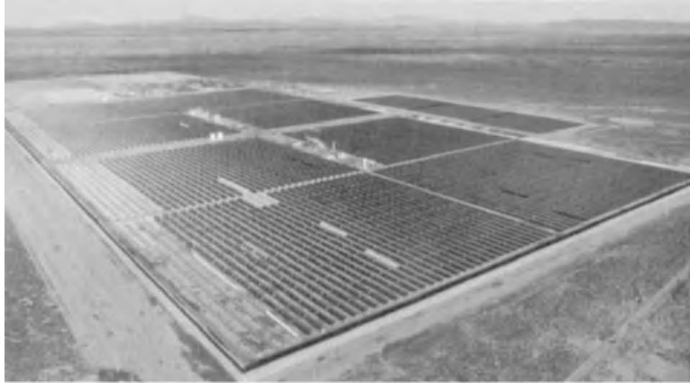
Figure 17.3.1 Aerial view of SEGS III, IV, and V, three of the Luz plants located on the Mojave Desert of southern California. Photo courtesy of Luz International, Inc.
