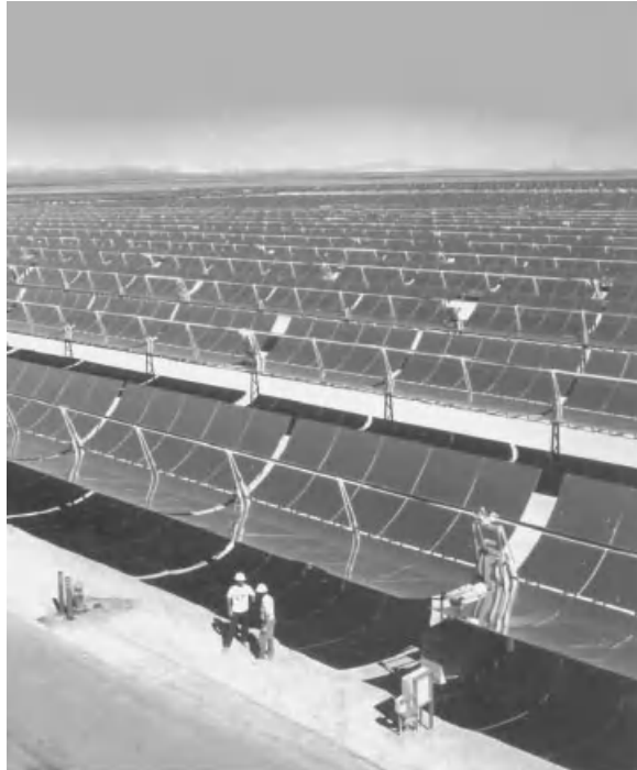
Figure 17.3.3 (a) SEGS collector fields.
