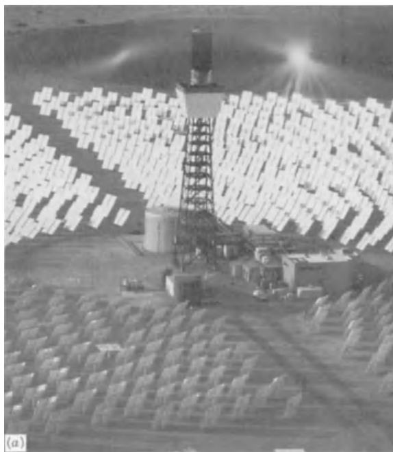
Figure 17.5.1 Solar One, at Barstow, CA. (a) Overall view of the heliostat field and receiver tower when system was not operating. (b) A heliostat. (c) The receiver, photographed from above, when in operation. Photographs courtesy of Sandia National Laboratories.
