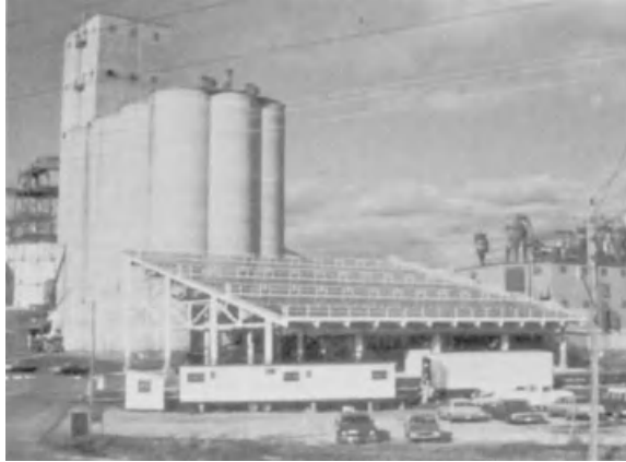
Figure 16.4.2 The 1200-m 2 air heating collector array at the Gold Kist soybean plant at Decatur, AL. Courtesy of Solaron Co.
