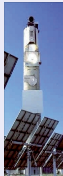
Helisotat Tower plant
