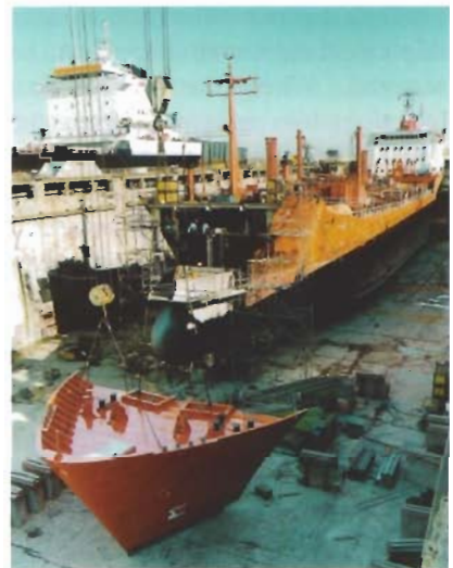
The bow brought in position.
