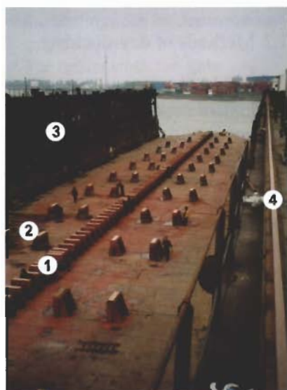
A floating dry-dock. Data: length = 217 metres, width (internal)= 32 metres, draught above blocks = 7.5 metres, lifting capacity = 25,000 tons.
