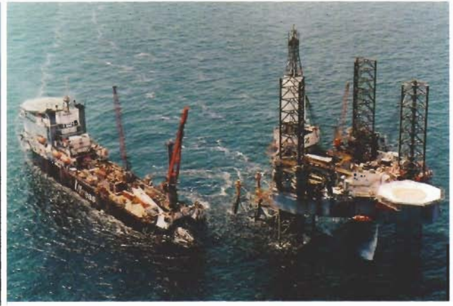
S-lay pipelaying vessel on DP working near a Jack-up platform
