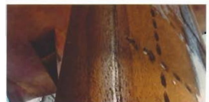
Cavitation damage on a rudder blade
