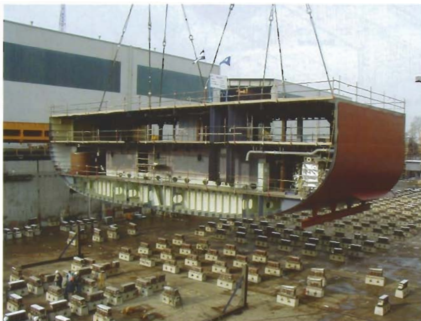
The first bottom segment is placed.
