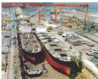
Construction in an excavated dock
