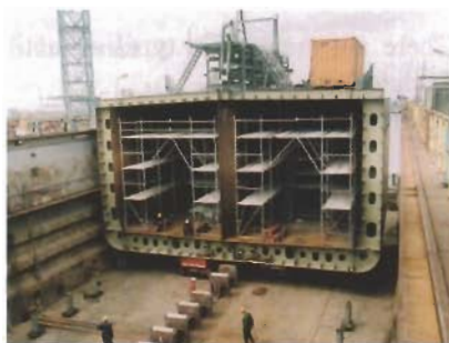
Tanker being built in a dry-dock
