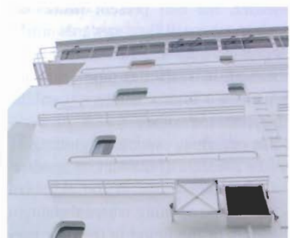
Ventilation grill for the accommodation
