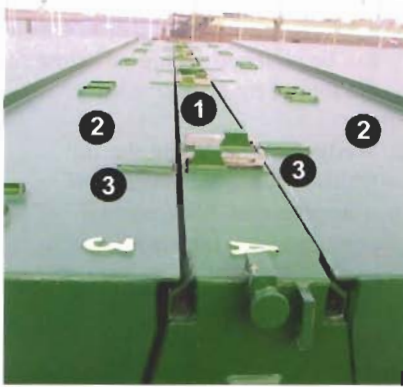
Beam between two closing hatches
