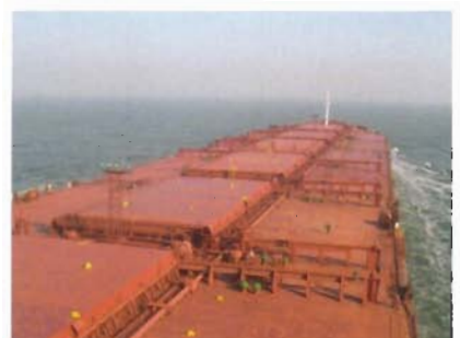
Bulk carrier. Every hatch to be closed with one hatch cover
