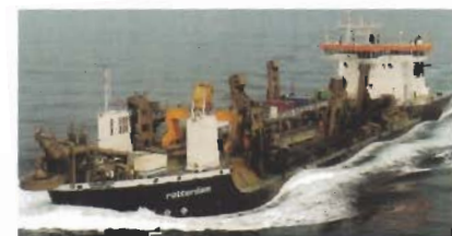
Trailing hopper suction dredger
