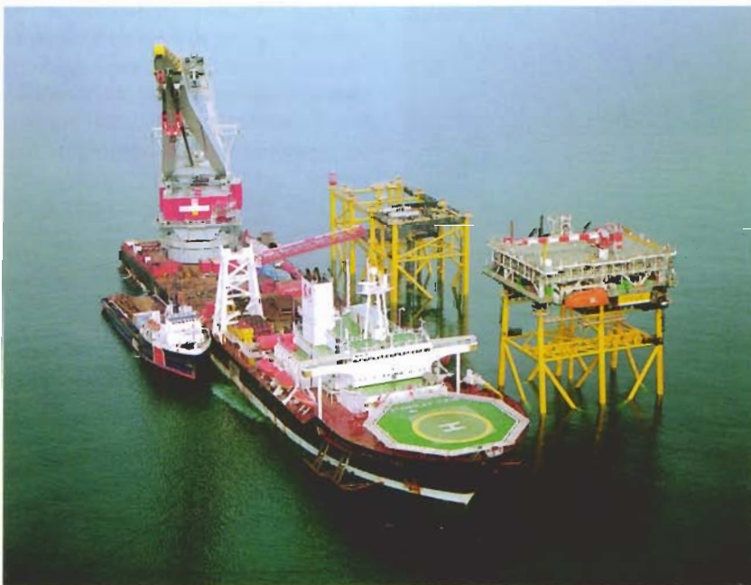
Crane vessel installing fixed platform
