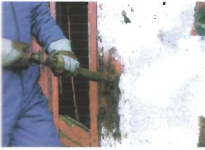
A pneumatic scaling hammer
