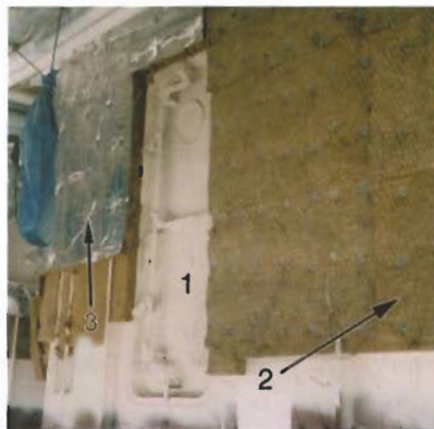
Part of accommodation insulated by glass wool on welding pins
