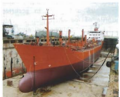
The new bow is attached
