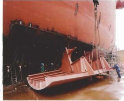
...and brought in position to be attached
