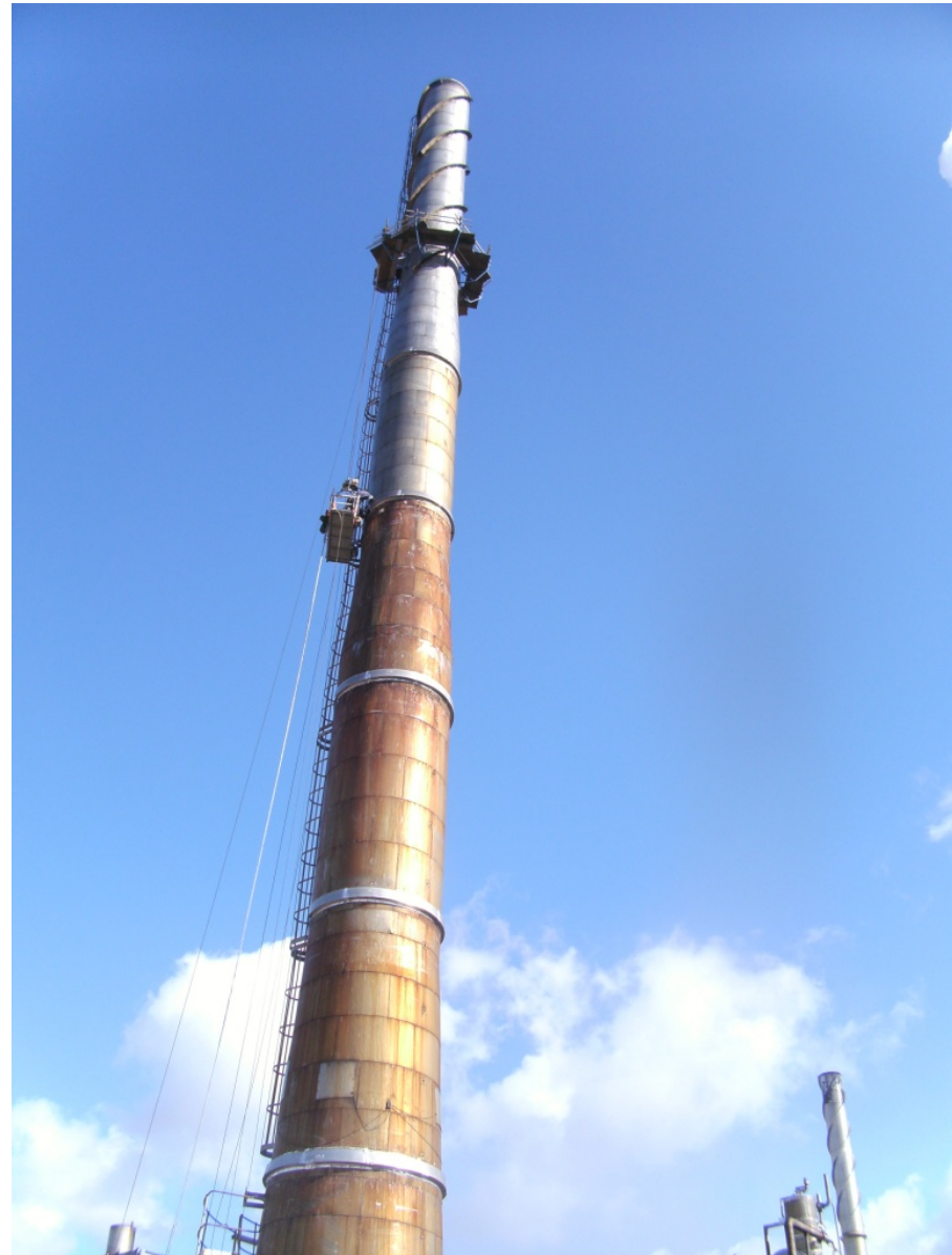
Steel chimney with helical strakes
