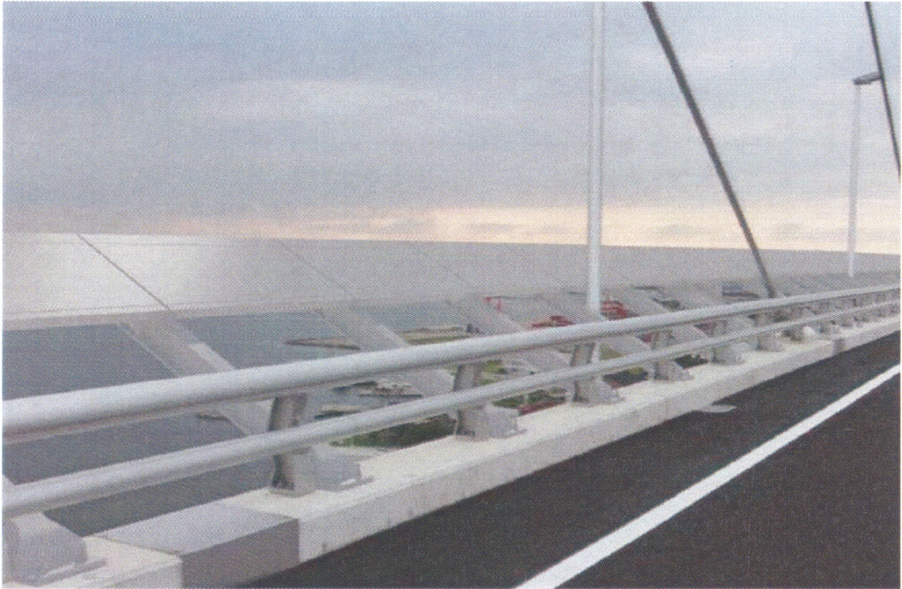
Cable-stayed bridge, Japan, equipped with flaps
