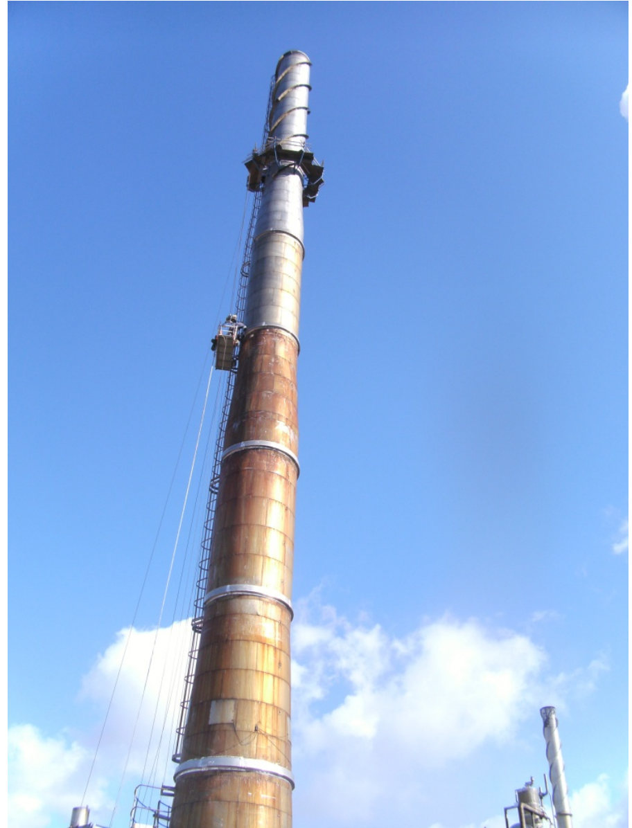
Stiffening rings for avoiding ovaling
