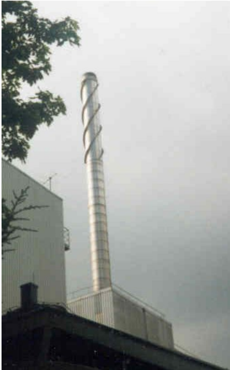
Steel chimney with helical strakes
