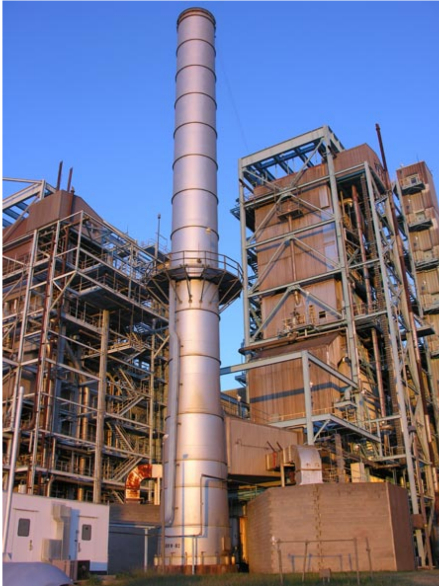
Stiffening rings for avoiding ovaling
