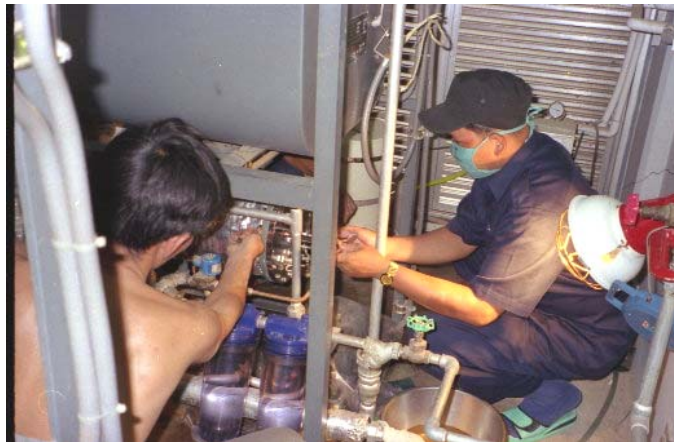
Photo 1.12 Preventive maintenance for a High-pressure Steam Steriliser (National Maternal and Child Health Centre, Cambodia): Two technicians carry out regular inspection and preventive repair to avoid equipment breakdown which would result in interrupting hospital function.
