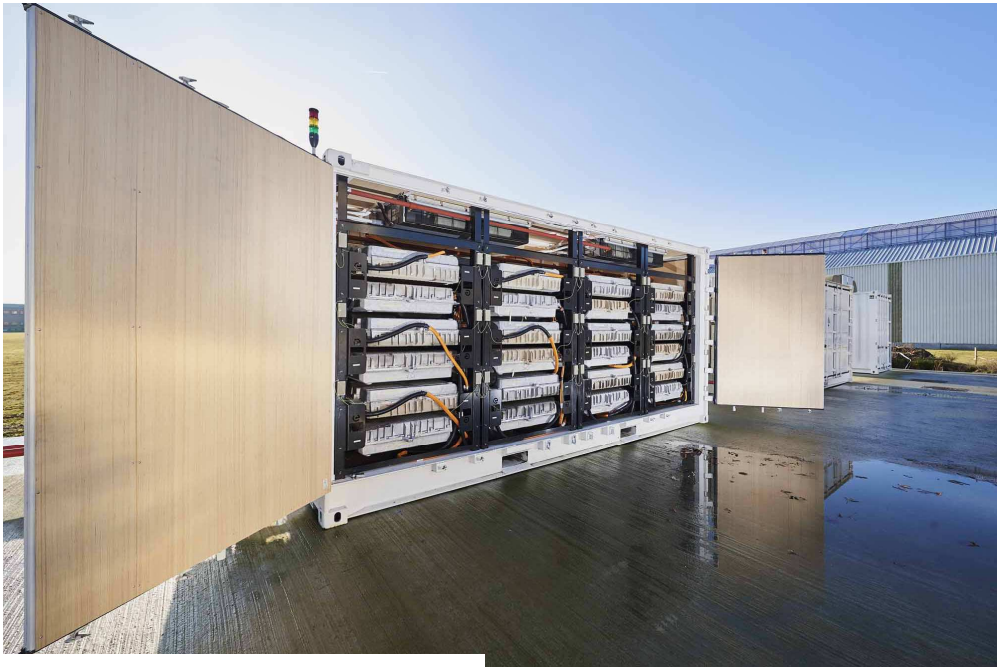
Second life batteries as stationary storage for Solar panels (Renault Group)
