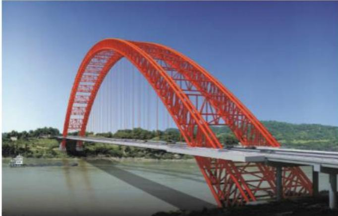
The longest CFST (Concrete Filled Steel Tube) arch bridge is the First Hejiang Yangtze River Bridge with a main span of 530m, 2013
