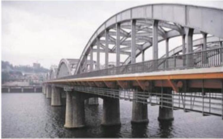
Figure 5: Han River Bridge (L=841m, arch portion 6x62.554m, B=20.3m, 1982)
