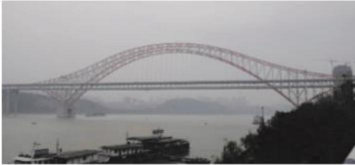
Chaotianmen Bridge with the world's longest main span of 552m in Chongqing (steel truss arch bridge, 2007)
