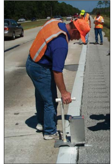
FIGURE 143 The Georgia Faultmeter in Use.
