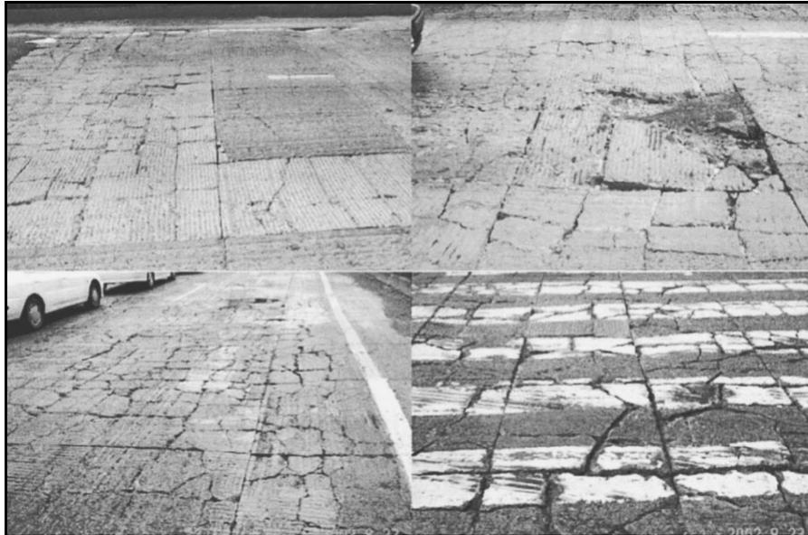
*Figure A.2. Severe distresses at 2 months for UTW projects in Taiwan [from Lin and Wang (2005)].*
