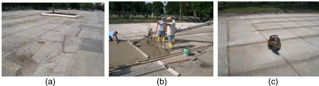
Figure A.1. Photographs of the E-15 parking lot (a) before, (b) during construction, and (c) saw-cutting pattern of the UTW.
