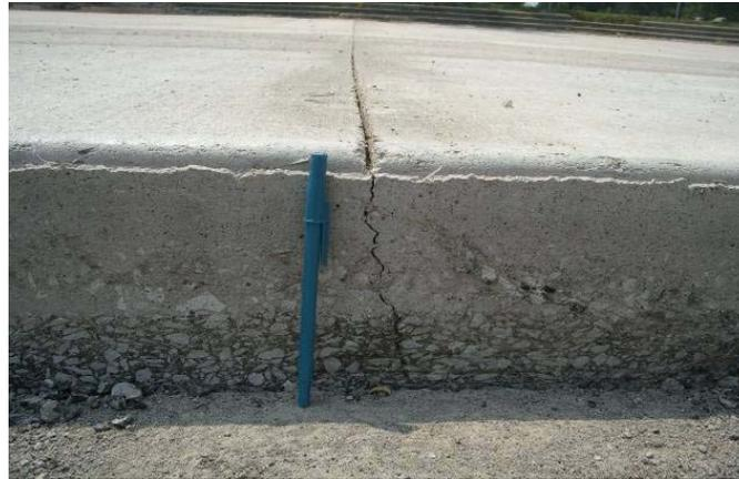
Figure B.22. Full-depth transverse joint crack through PCC and HMA layers.
