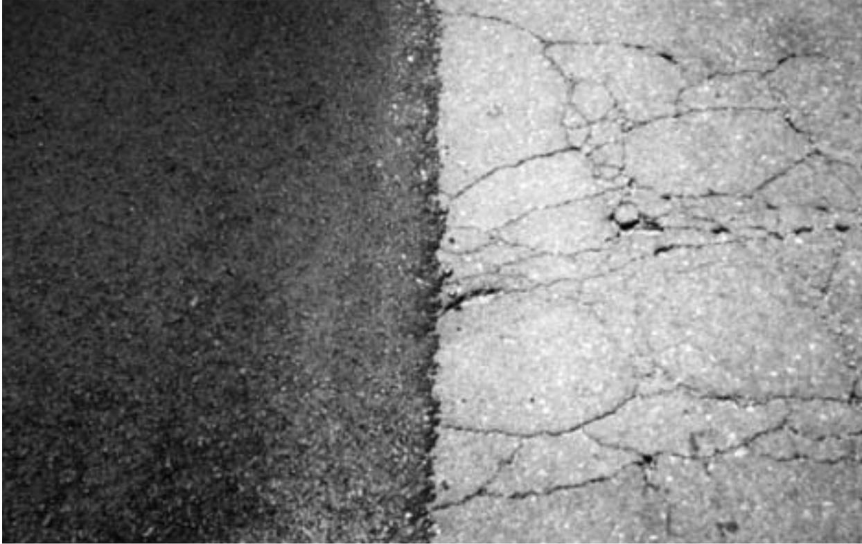
*Figure 6-10: Surface Recycling before and after*
