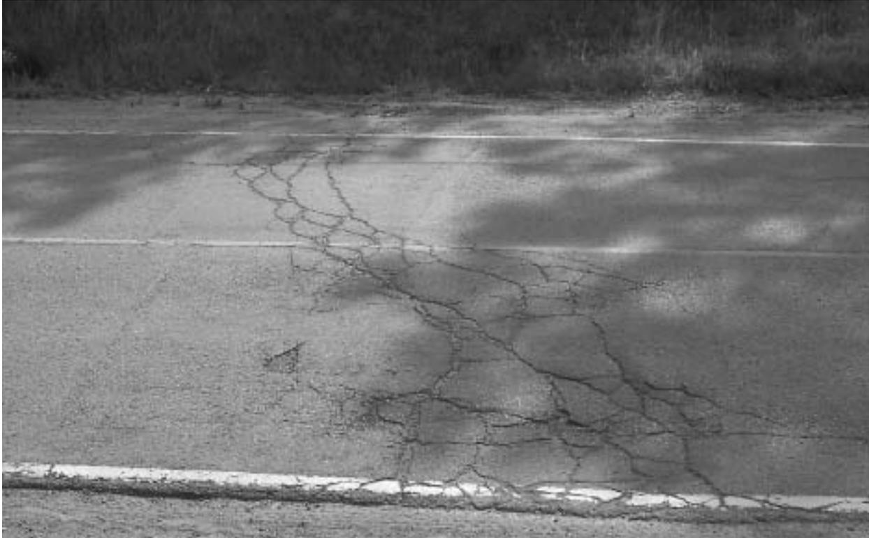
*Figure 3-2: Cracking Distress*
