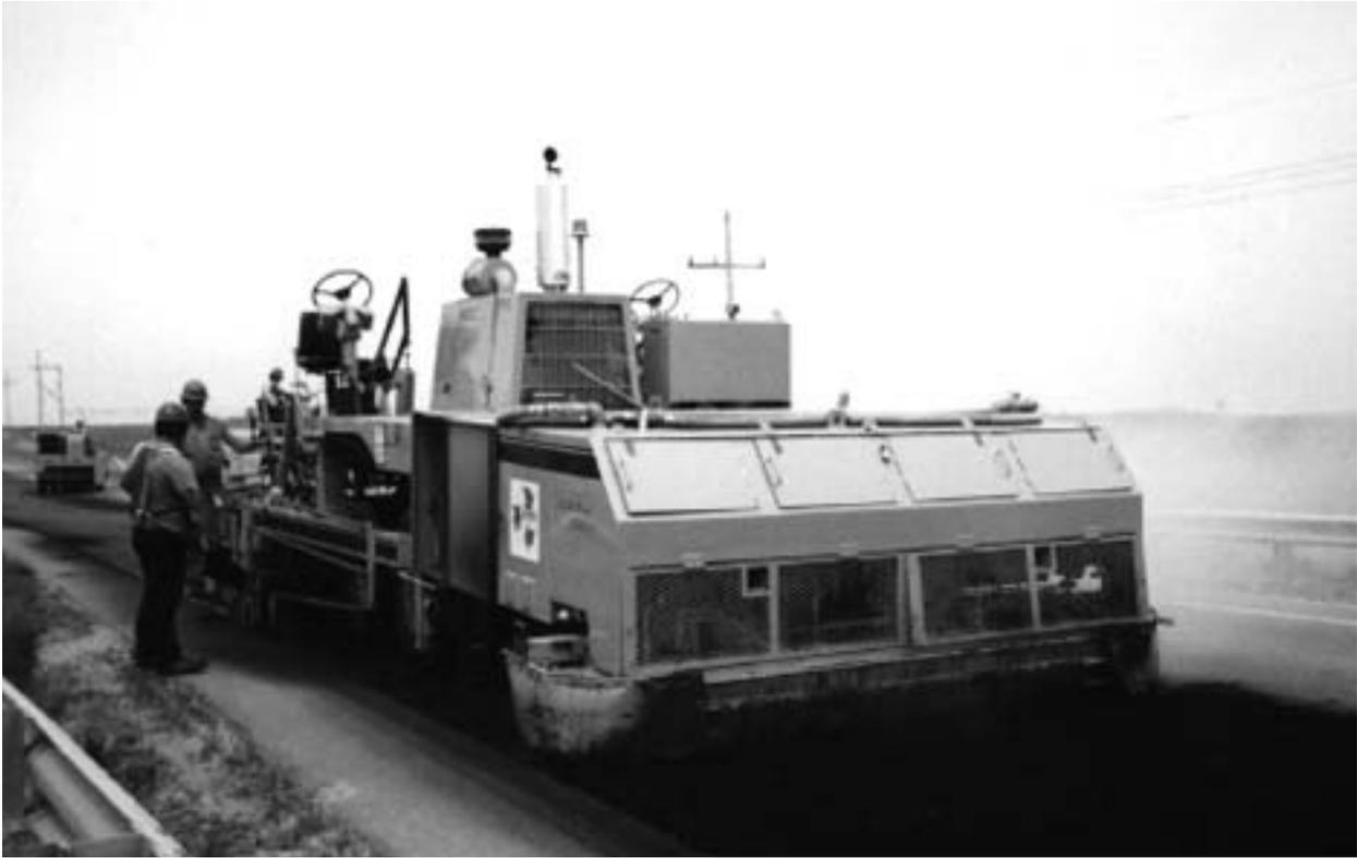
*Figure 6-5: Recycling agent addition, mixing, and paving unit*
