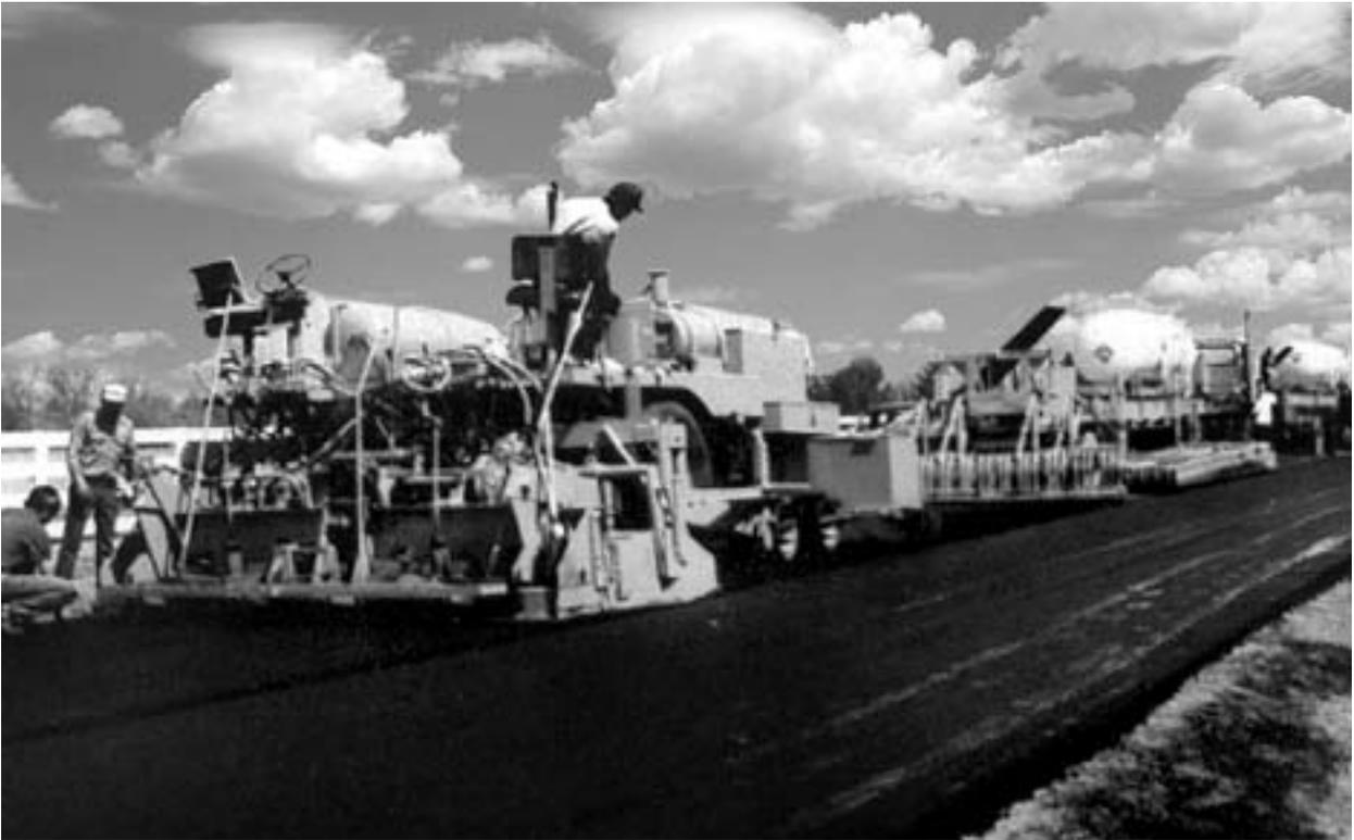
*Figure 1-9: Recycled mix placement*
