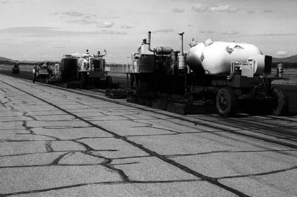
*Figure 1-7: Surface Recycling heating units*
