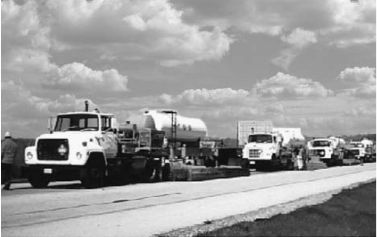
*Figure 6-1: Surface Recycling preheaters*
