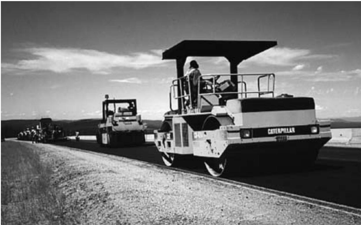
*Figure 6-19: Compaction of recycled mix*
