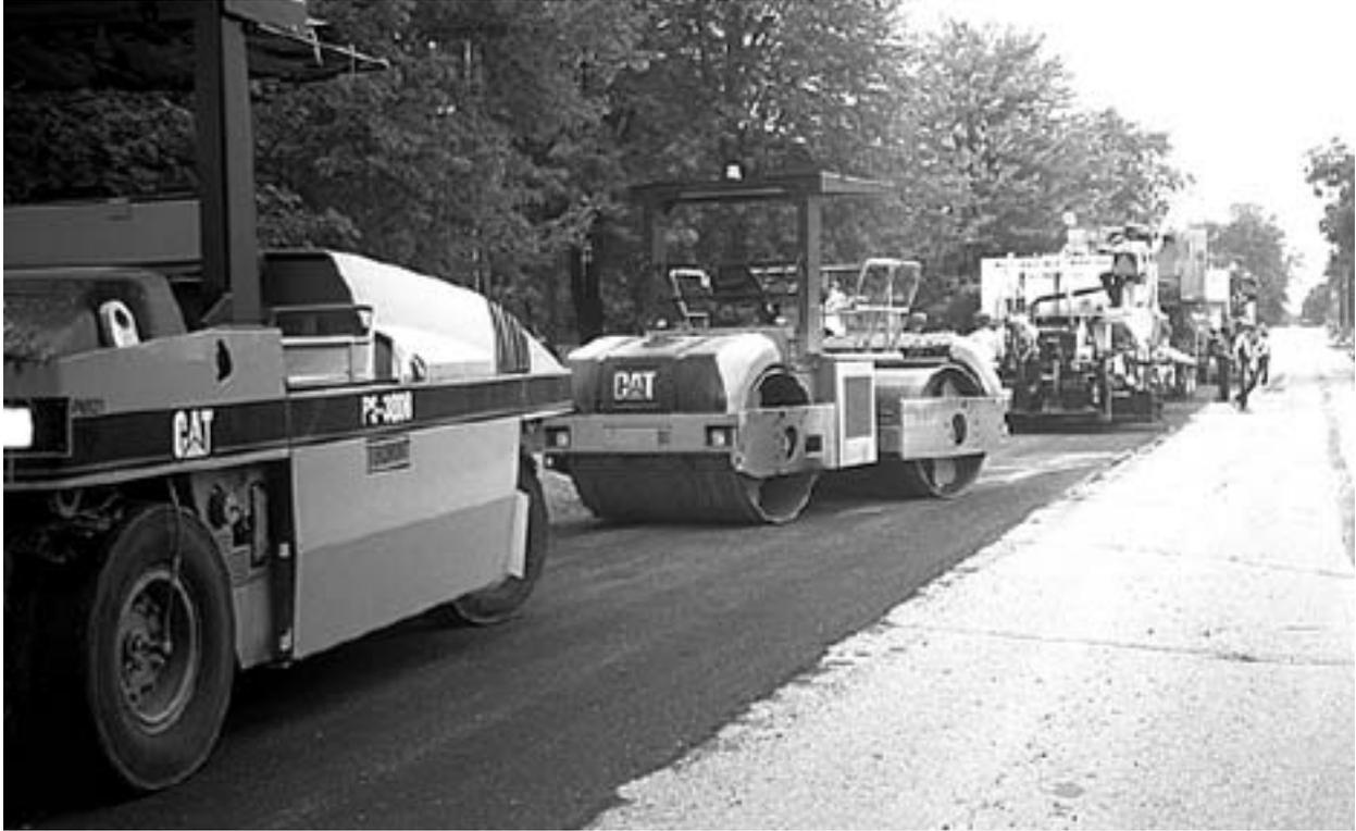
*Figure 1-21: CIR compaction*
