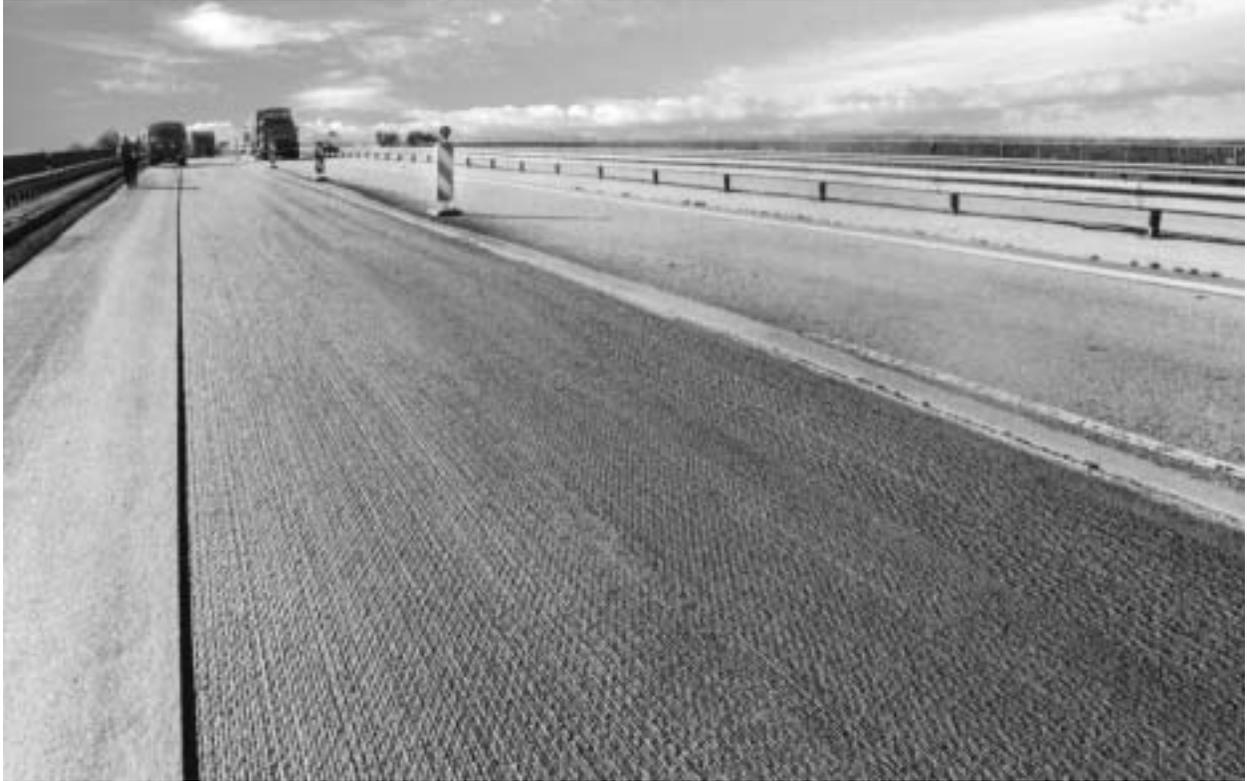
*Figure 1-3: Milled pavement surface texture improve friction numbers*
