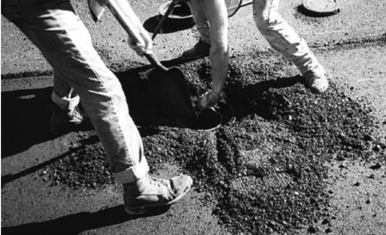
*Figure 6-18: Raising water valve after remixing*
