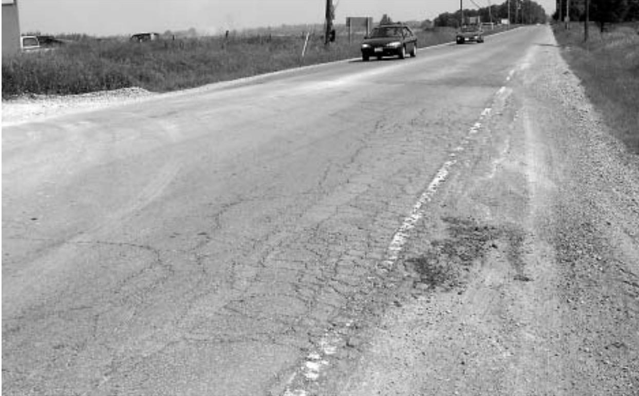
*Figure 2-4: Candidate Road for Rehabilitation Treatment*
