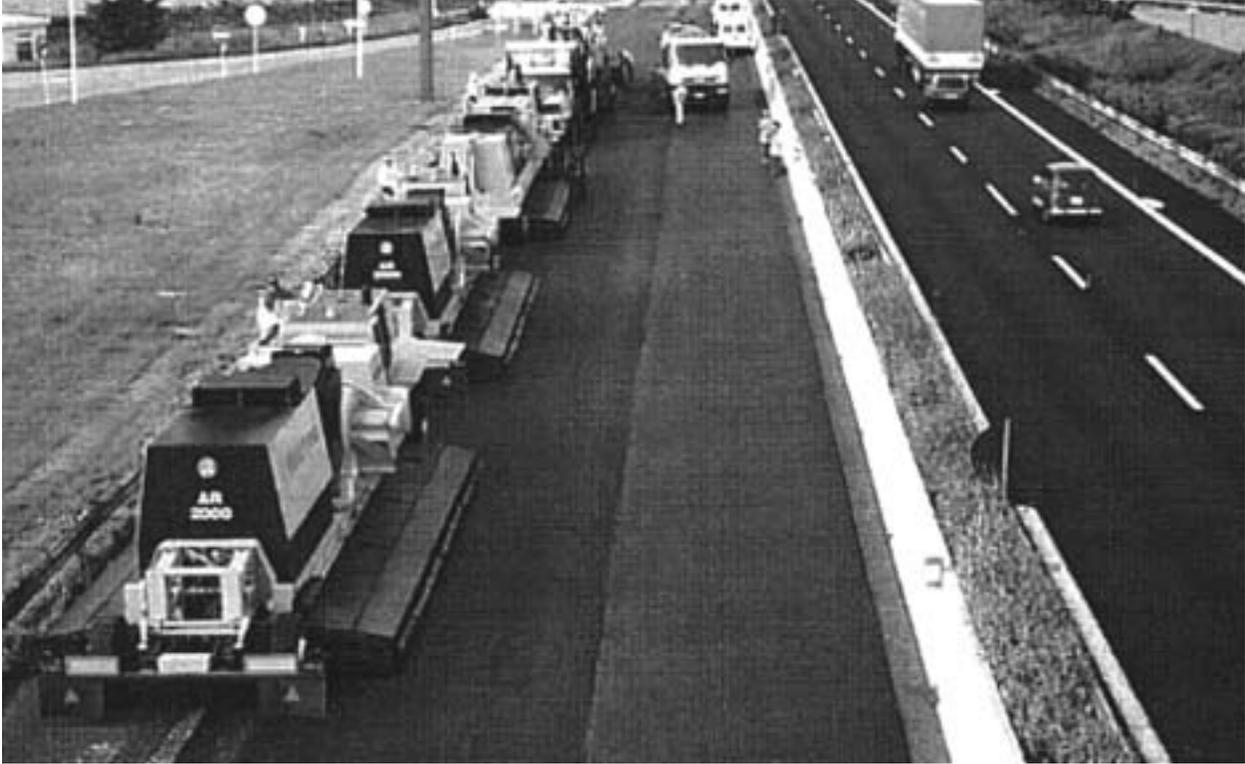
*Figure 6-11: Single stage Remixing train*
