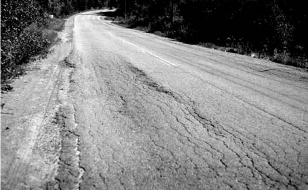
*Figure 3-3: Base and Sub-Base Deficiencies*
