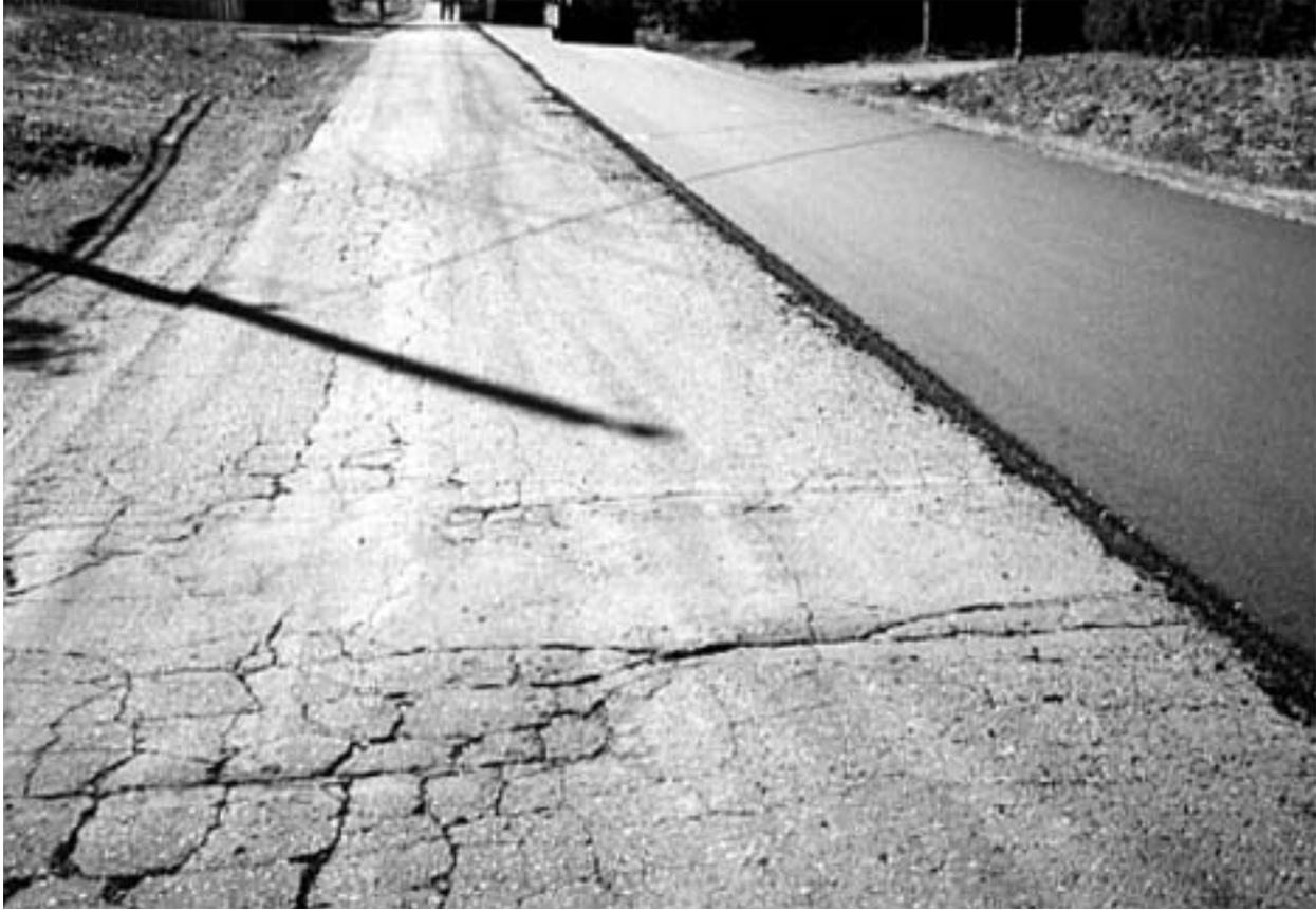
*Figure 6-23: HIR Repave before and after*
