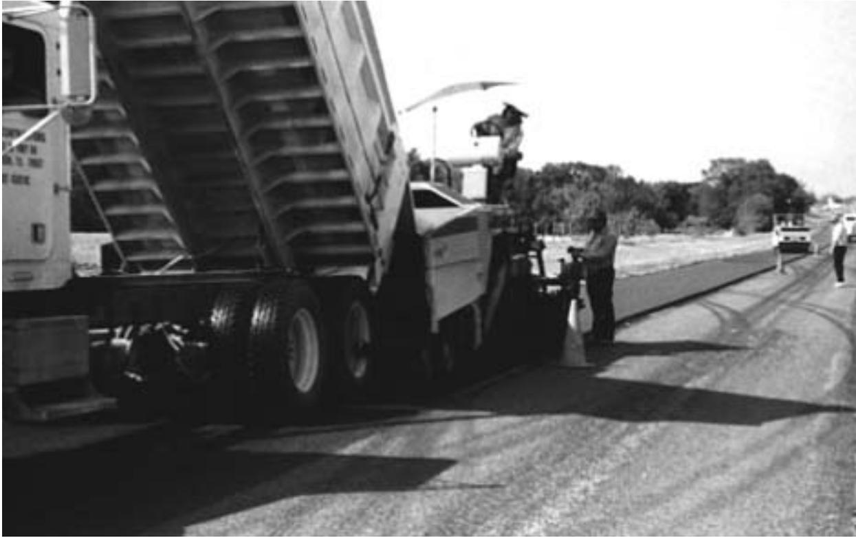
*Figure 1-24: CCPR mix placement*
