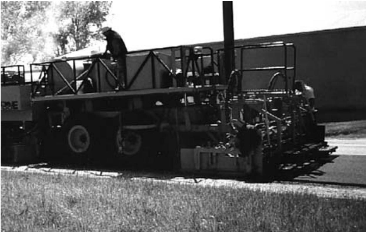
*Figure 6-16: Remixing unit and integrated screed*
