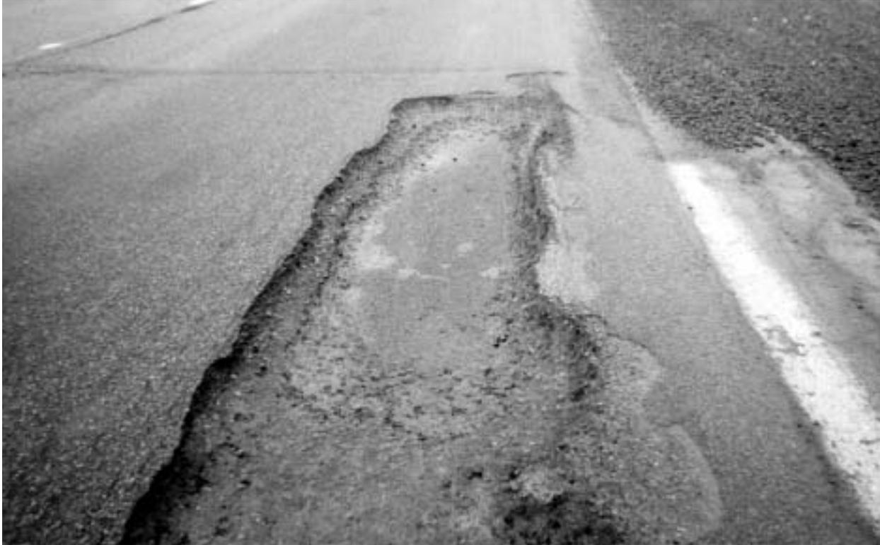
*Figure 3-1: Pothole Pavement*
