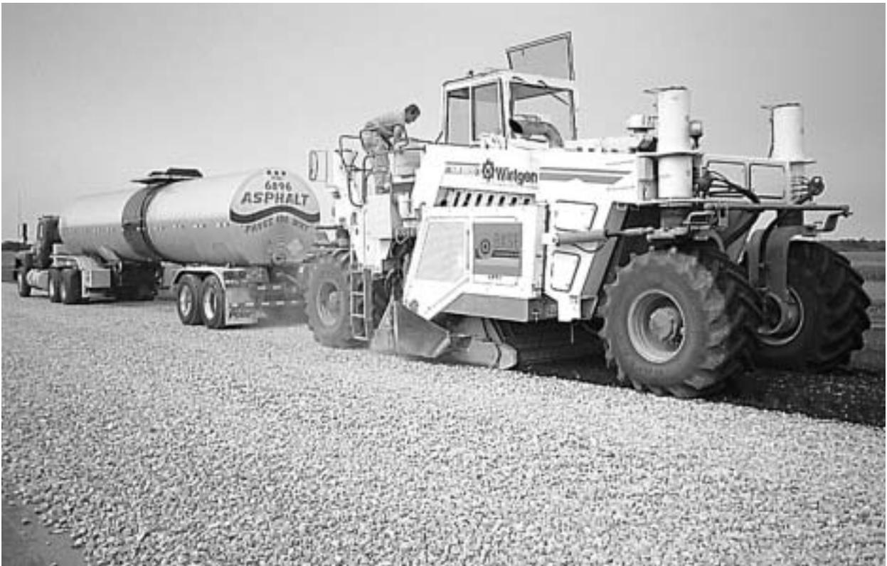
*Figure 1-16: FDR reclaimer and stabilizing additive tanker*
