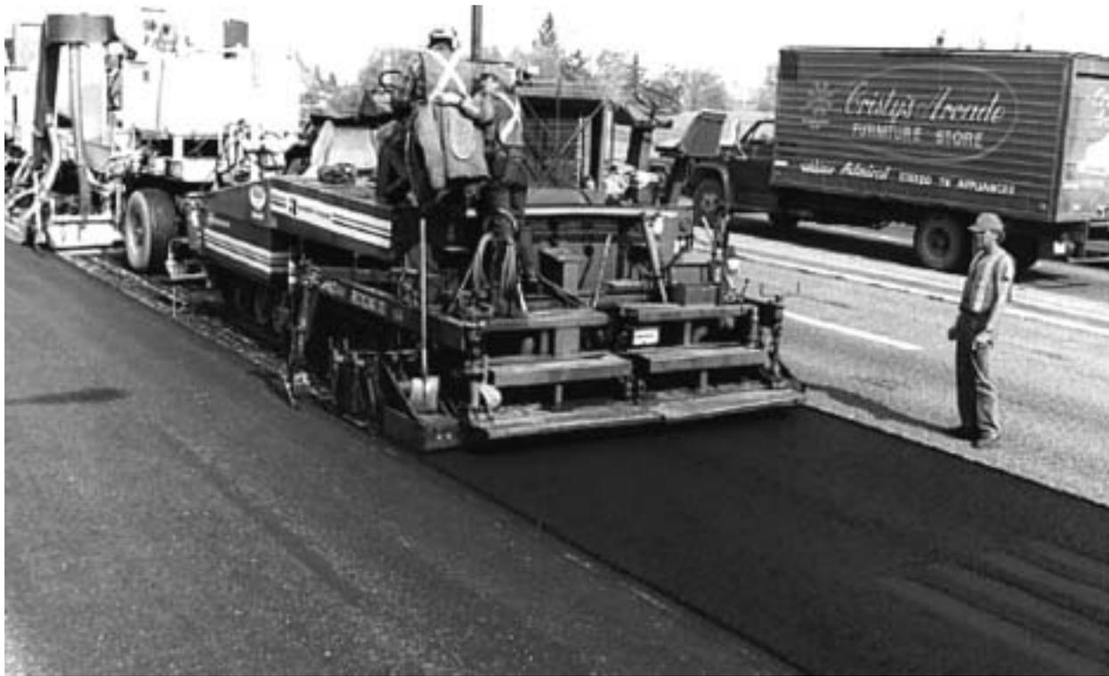
*Figure 6-17: Conventional HMA paver placing recycled mix*
