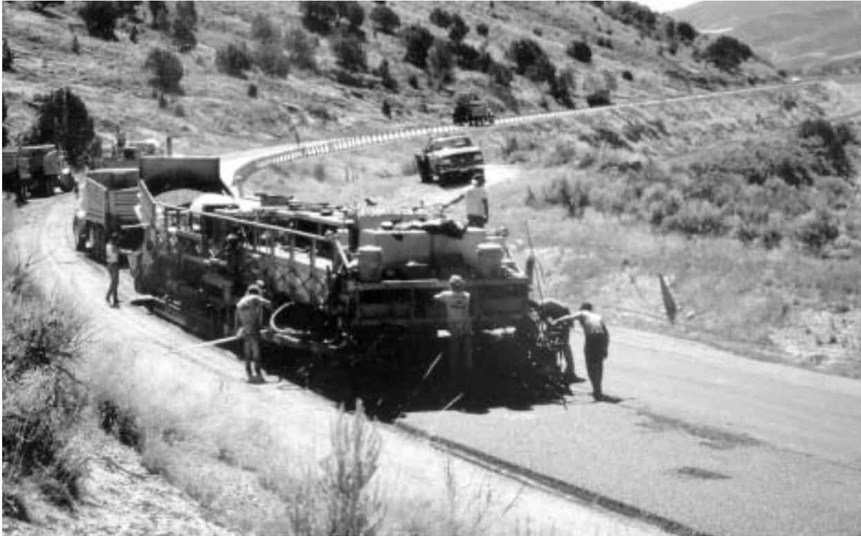
*Figure 1-14: Single pass repaving*
