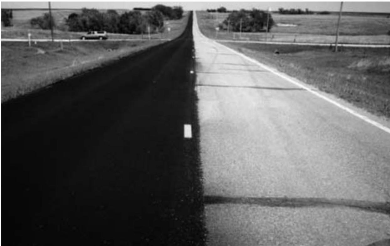
*Figure 6-9: Surface Recycling before and after*
