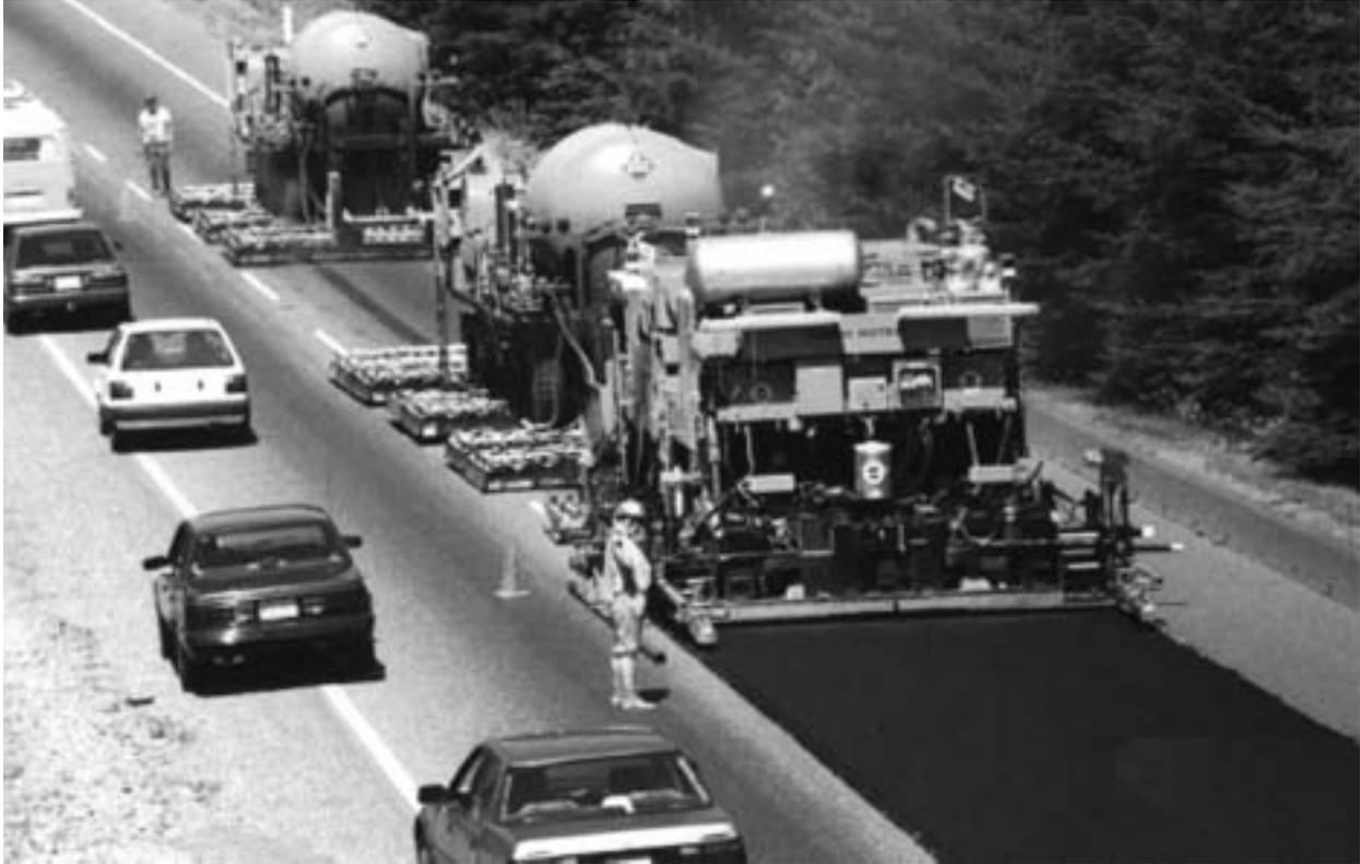
*Figure 1-11: Single stage Remixing train*
