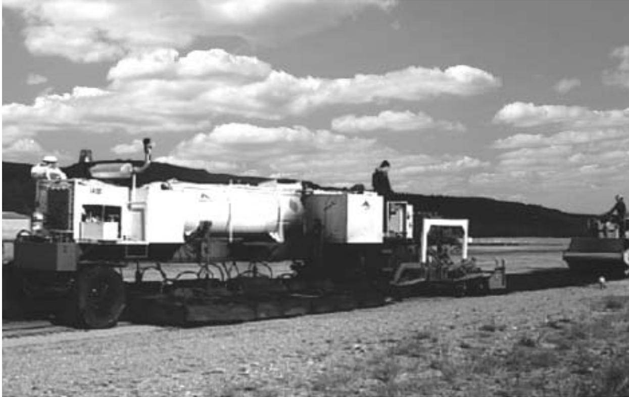
*Figure 6-7: Free floating screed on scarification unit*
