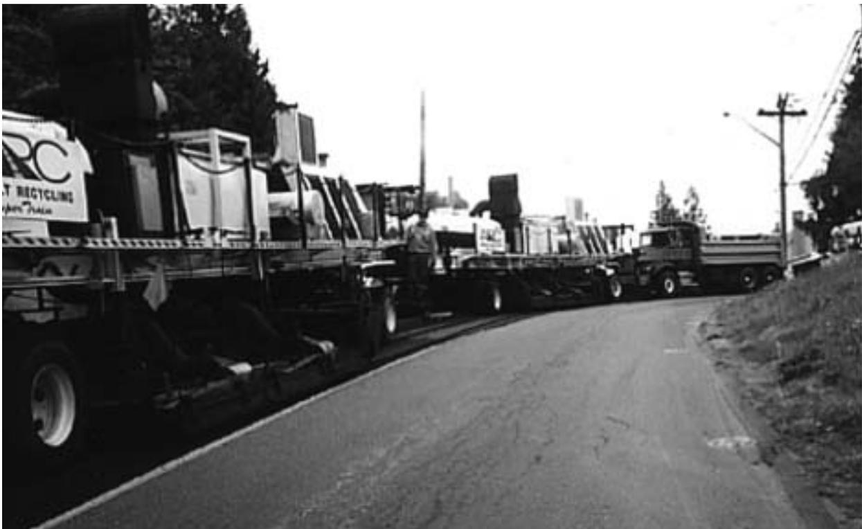
*Figure 6-12: Multiple stage Remixing train*
