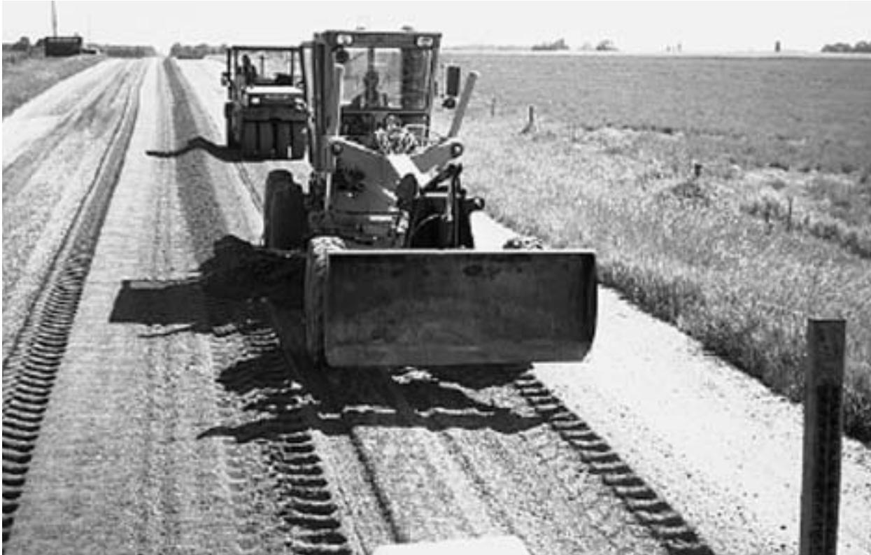
*Figure 1-17: Initial shaping with motor grader and compaction*
